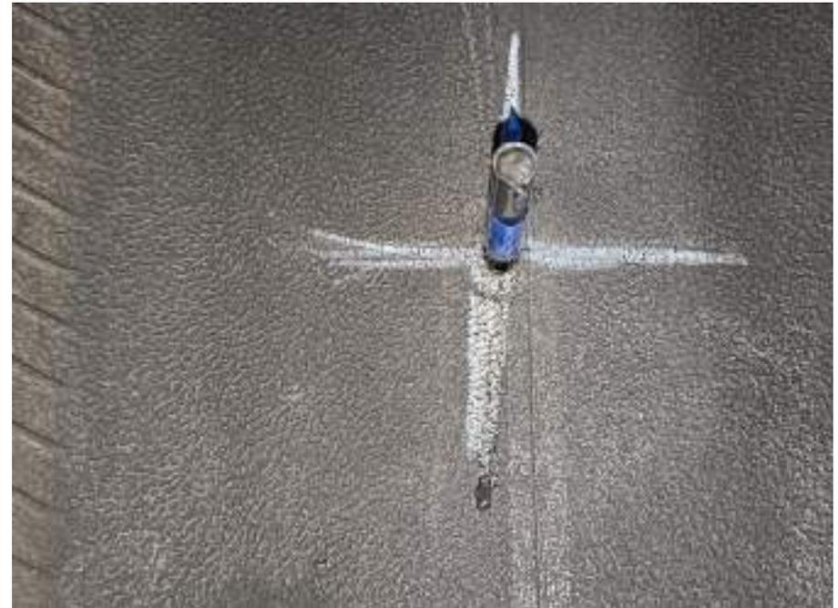
**Guide the Plug into the injury using the guide wire. Once it is positioned in the injury remove the poly film**
