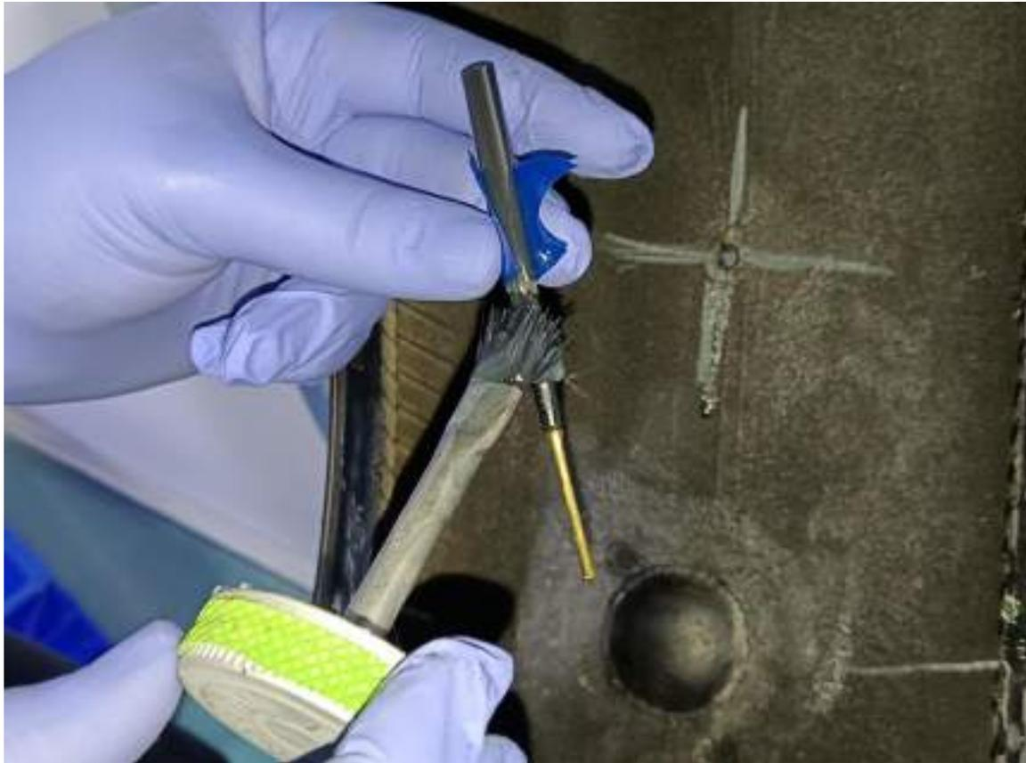
**Apply one coat of Fast Dry Cement or CVF on the stem of the Stem Plug patch.**
