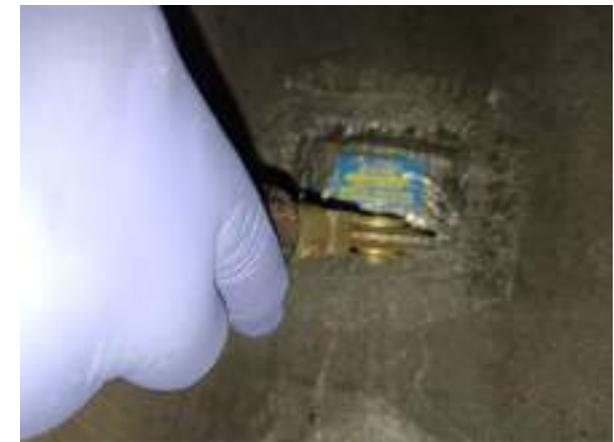
**Stitch the patch from the center to either sides vigorously using a serrated hand Sticher.**
